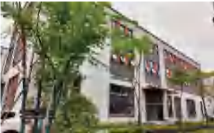
Chongqing Bishan Production and Processing Base (Sino-American Joint Venture)
